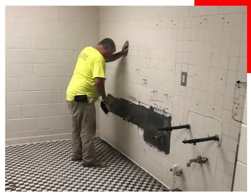
Mason Refacing Block in 8<sup>th</sup> Street Group Bathrooms for new Ceramic Wall Tile
